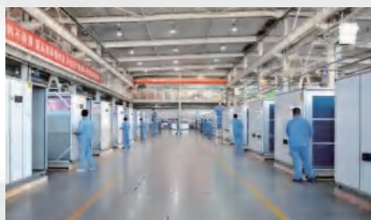
Assembly area of combined air handling unit
