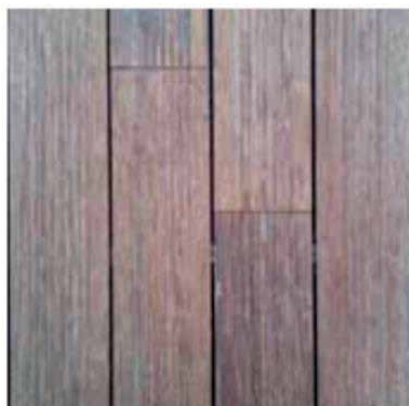
Weathered but cleaned flooring
