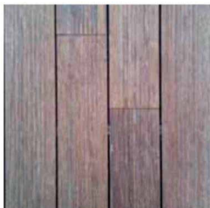
Weathered but cleaned flooring
