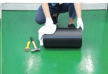
② Clean the pipe
