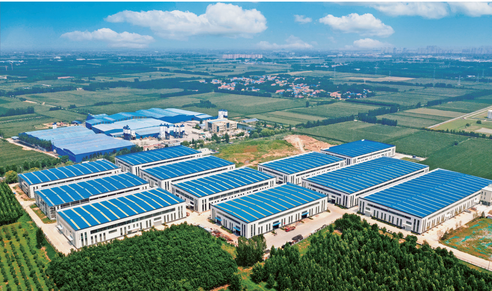
Shandong Fuding Industrial Park
