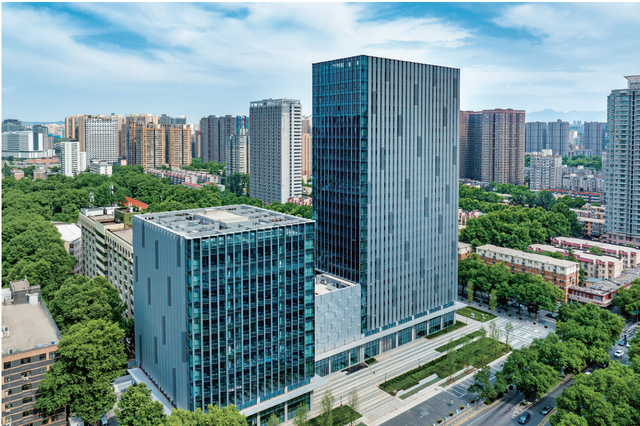
Training building of Xi'an University of Architecture and Technology
