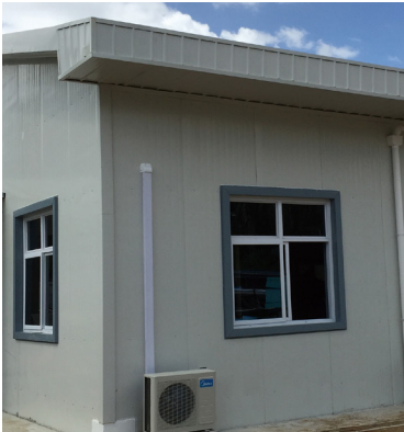
Suriname Ministry of Foreign Affairs Office Building Project
