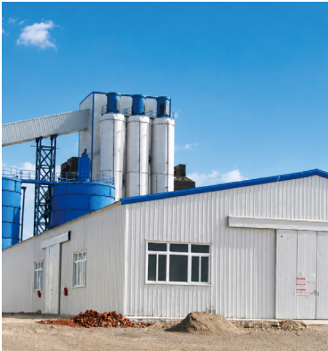
Upper Atbara Hydropower Plant Warehouse Project in Sudan
