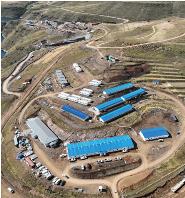
Lesotho Water Conveyance Tunnel Project
