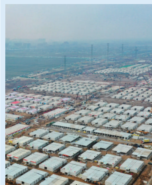
Shijiazhuang Isolation Center Project
