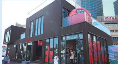
The 5A-level scenic area project on the west bank the Tongzhou Canal
