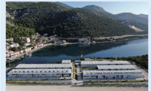
The China Road and Bridge Corporation Croatia Cross-sea Bridge Camp Project
