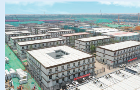
The Beijing Urban Construction Xiongan Builders' Home Project
