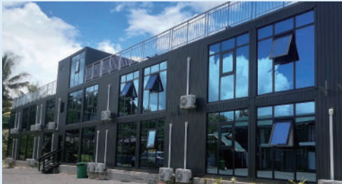
Samoa modular container house hotel project
